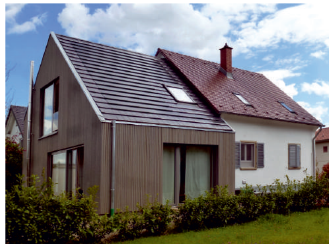
3 solar roof panels cover an area of approx. 1 m 2 , weight approx. 24 kg. Nominal output of 14 solar roof panels approx. 1.05 kW.
