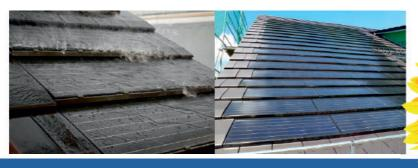
No penetration of the roof cladding and insulation e.g. through the screw connections of roof hooks
